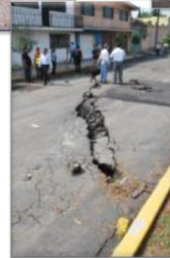
Tensional open fracture without significant vertical displacement
