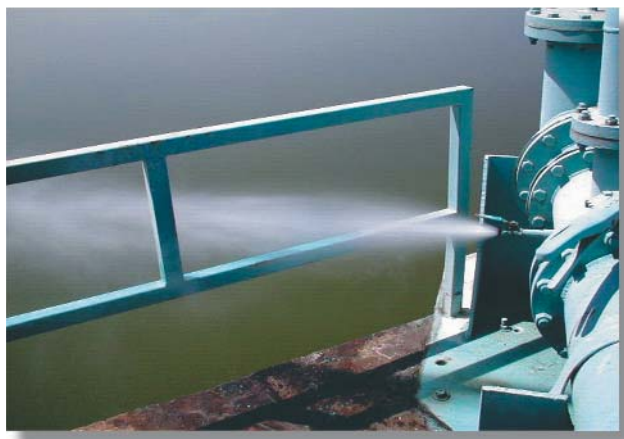
AIR CONTENT IN WELL WATER FROM THE PEÑÓN-TEXCOCO BRANCH IN THE STATE OF MEXICO
