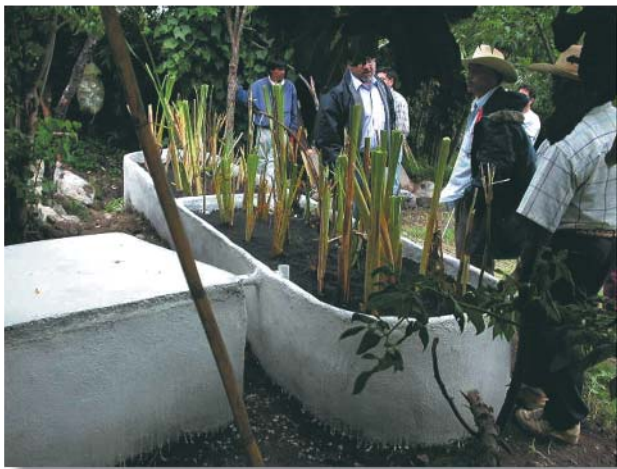
THE WORKSHOP CONSTRUCTION OF A BIOFILTER: HOME GRAYWATER TREATMENT IN THE COMMUNITY OF SAN JERÓNIMO PURÉCHECUARO, QUIROGA, MICHOACÁN
